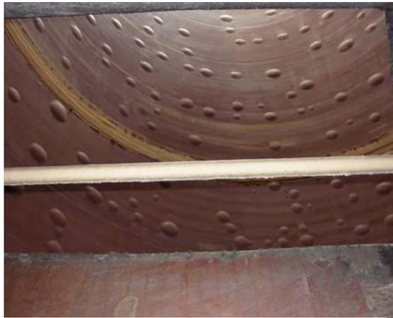
**Image 2.3: Bigger blisters in a flue gas duct**
