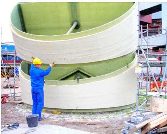
Image 6.2: Pre-assembly of a 17'Ø mitered elbow
