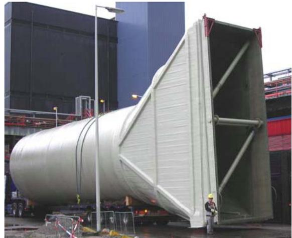
Image 6.3: Insulated 17'Ø flue gas duct section, connected to 10'x30' breaching
