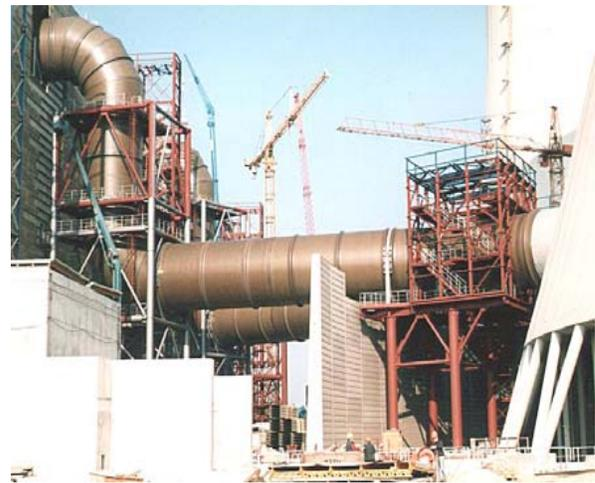
Image 1.2: Flue gas duct (21'-4"Ø) at Schwarze Pumpe
