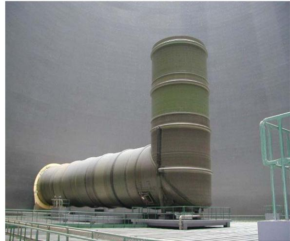
Image 1.1: Flue gas duct (23'-0"Ø) in a brown coal plant at Florina (inside of cooling tower)
