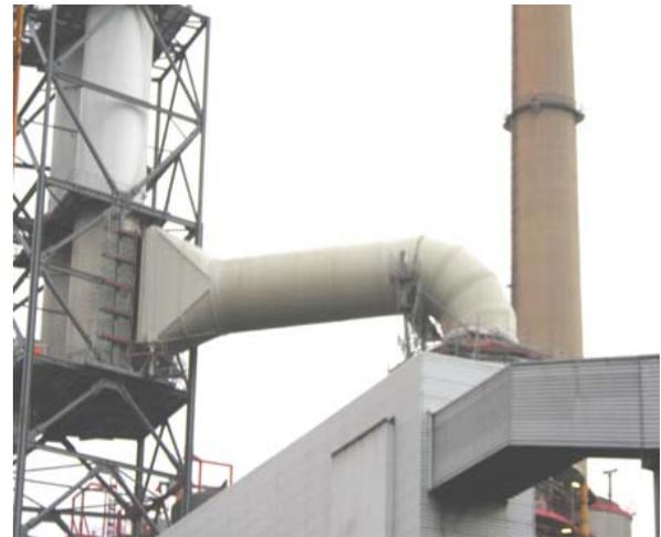
Image 6.4: Assembled FRP flue gas duct with the breaching connection to chimney
